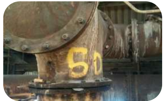
Cold bond steel plate to seal leaking pipe surfaces
