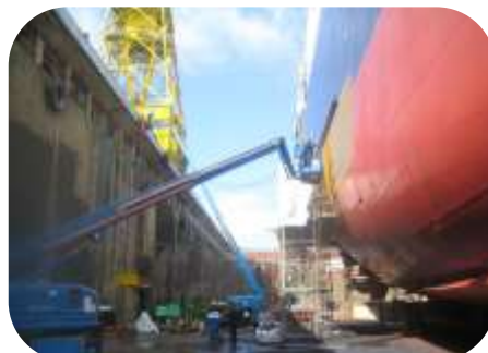
Corroded bow on large container vessel abrasive blast cleaned and filled using 101 Metal Repair Paste
