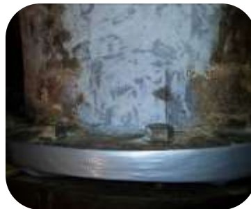
Cold bond steel plate to seal leaking pipe surfaces
