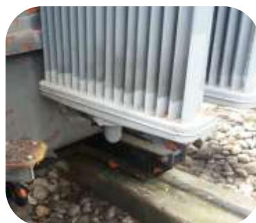
Weeping transformer surfaces manually abraded and sealed using 104 Metal Repair Fluid XF
