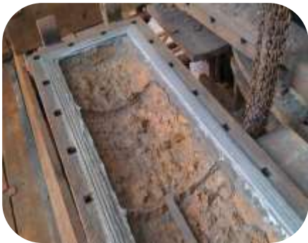
Seal on a process vessel door had been badly corroded from chemical attack. The seal surface was re-formed using 101 Metal Repair Paste
